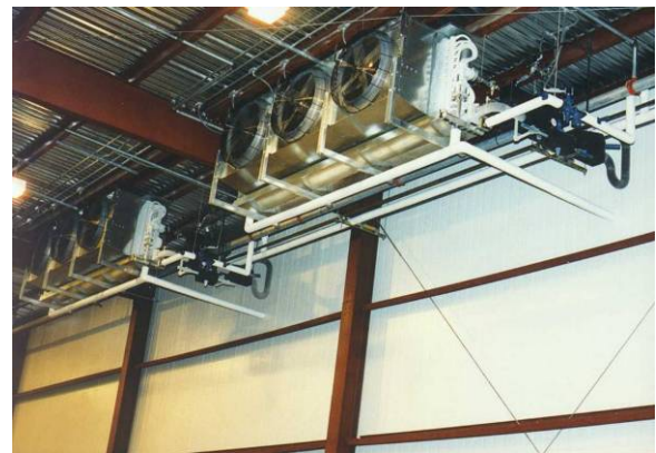
Typical warehouse application.
