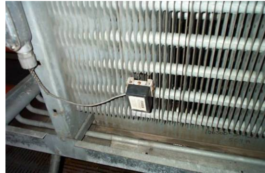
Sample evaporator frost sensor.
