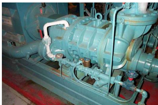
Sample liquid injection cooling.
