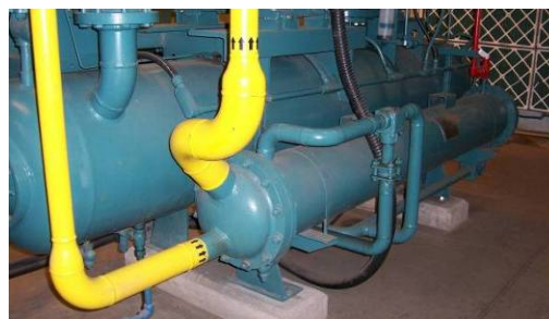
Sample thermosiphon application.
