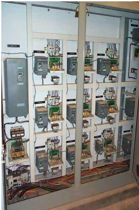
Sample evaporator fan VFD application.
