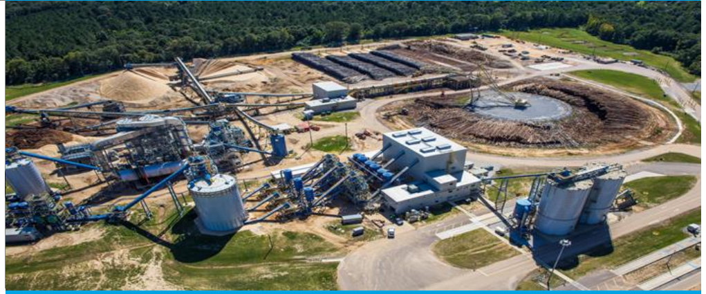
Aerial view of Amite Bioenergy in Gloster, Mississippi. Photo from Drax, retrieved from https://southerlymag.org .
